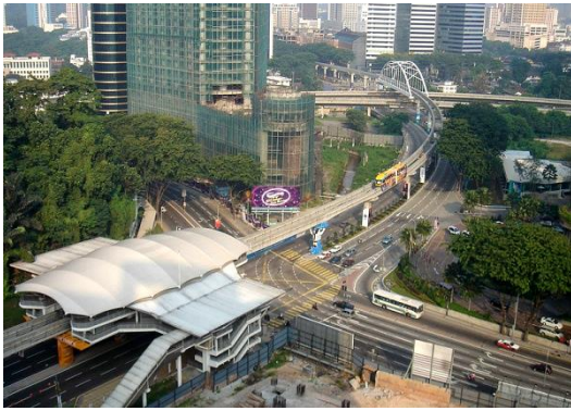
Figure 1.1: Integrated Public Transportation between LRT and bus in Kuala Lumpur (Source:en.wikipedia.org/wiki/Public_transport_in_Kuala_Lumpur: Sept 2012).
