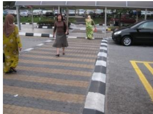
Figure 8.26: Flat-top speed hump doubling as pedestrian crossing at Bandar Tasek Selatan LRT station, Kuala Lumpur (Source: Muhammad Zaly Shah)
