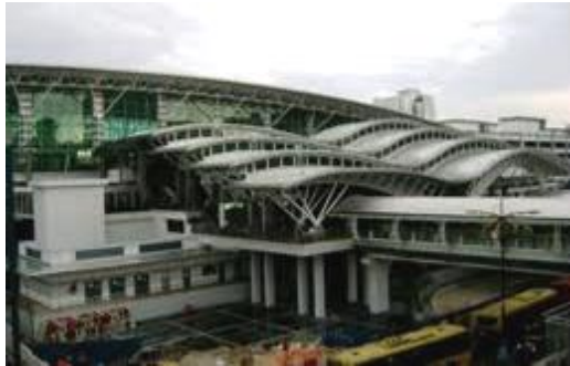
Figure 1.12: JB Sentral’s railway station and public transit station (Source: http://www.skyscrapercity.com :Sept 2012)
