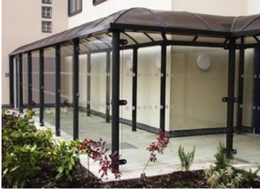
Figure 8.9: Covered walkways creating external corridors
