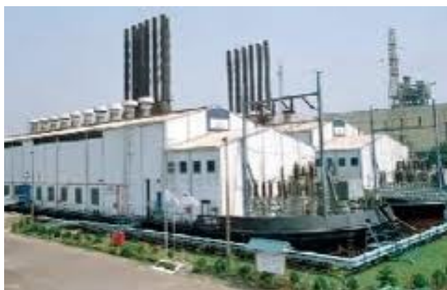
Fig. 12: Khulna Power plant
