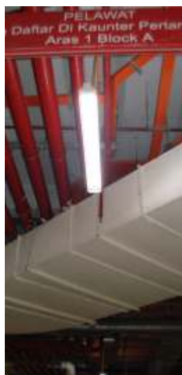
T6 fluorescent light fixtures are widely used in the basement parking area
